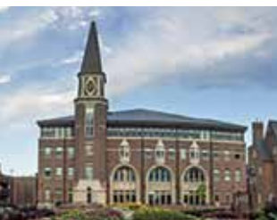
TOP TO BOTTOM Children's Hospital of Wisconsin
